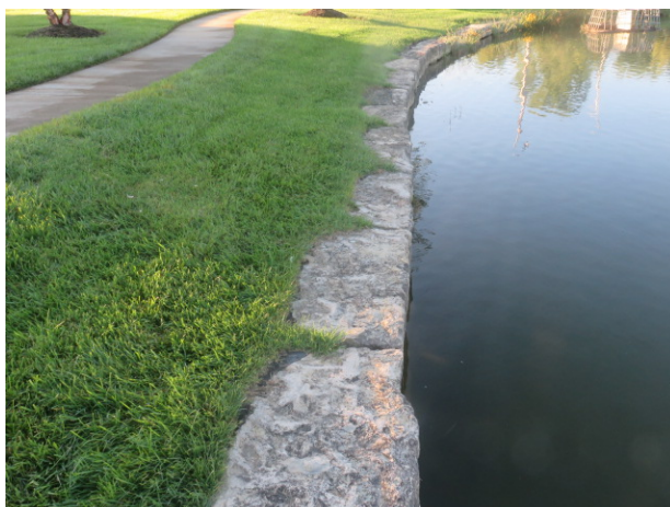
Section of shoreline with stone bulkhead
