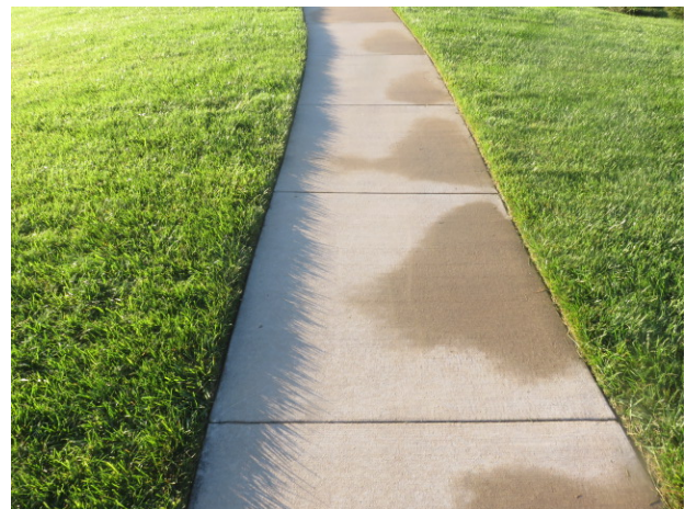
Concrete sidewalk in good overall condition
