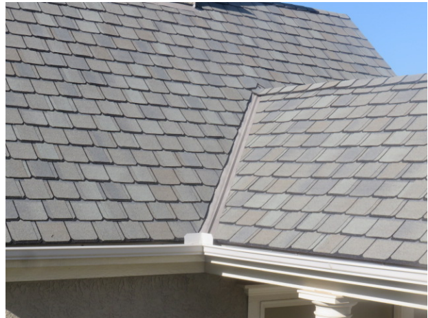
Open valley with w-flashing and adjacent gutters in good condition
