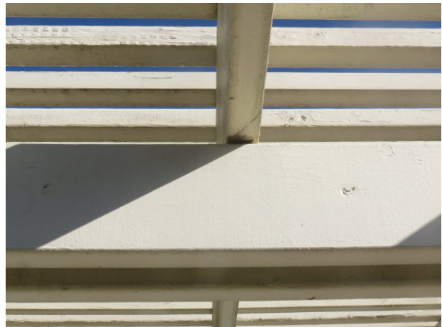
Trellis wood components in good condition
