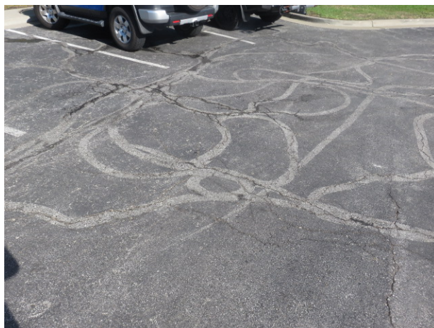
Repaired and unrepaired cracks at parking area Repaired and unrepaired cracks at parking area
