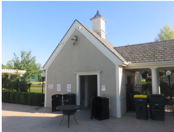
Stucco finish walls at the pool house
