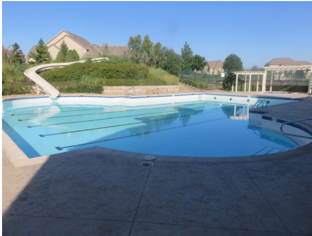
Main pool and deck overview
