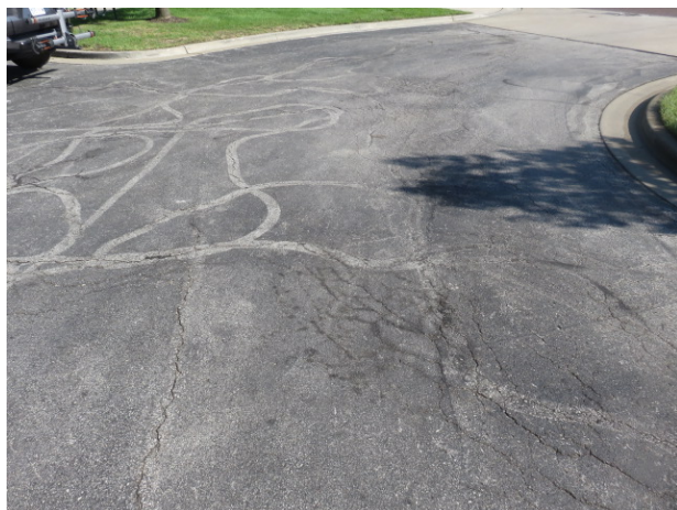
Repaired and unrepaired cracks at parking area Repaired and unrepaired cracks at parking area
