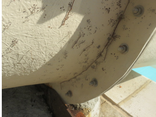
Underside view of slide and fasteners in good condition
