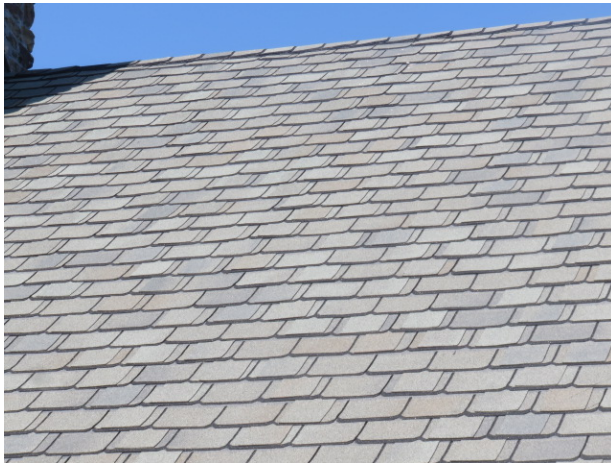
Asphalt shingles in good condition
