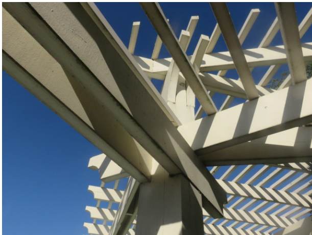
Trellis wood components in good condition
