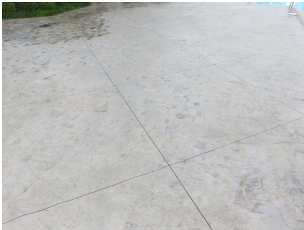
Concrete pool deck
