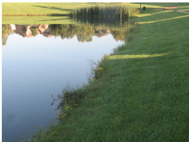
Isolated and minor instances of erosion
