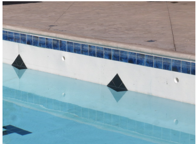
Plaster and tile pool finish
