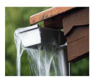
Clogged gutters will begin to hold water. Between the mounting water and the weight of the debris, gutters will become incredibly heavy. This can lead to the gutter breaking away from the fascia causing damage to this portion of the roofing system.
