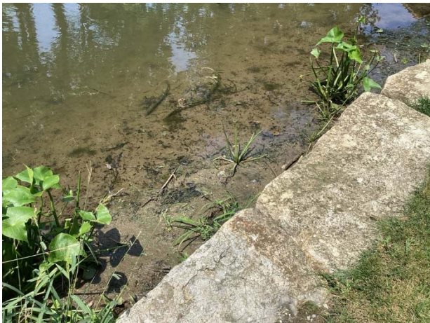
Sediment accumulation at north pond
