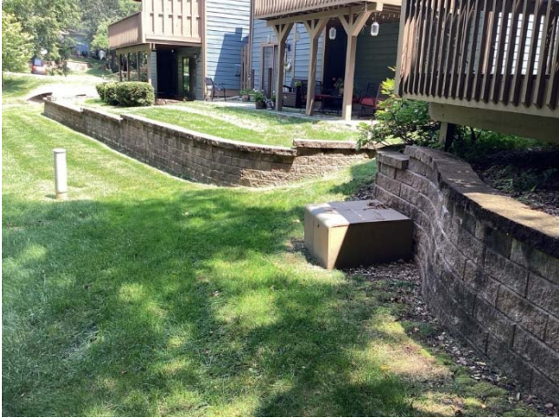
Masonry retaining walls behind homes at Lakeside Dr, note efflorescence
