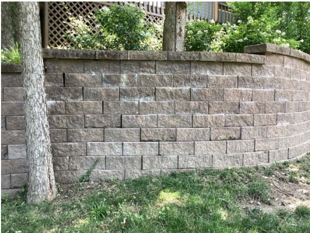
Efflorescence and wall displacement between trees at Lakeside Ct
