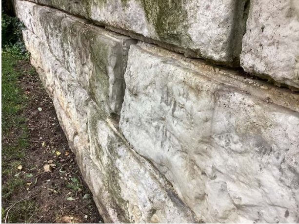
Isolated, minor displacement
