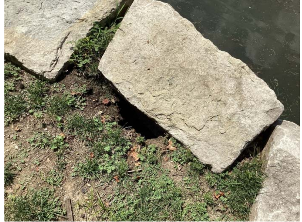
Erosion at wall backside
