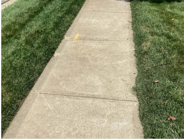
Sidewalk spalls and cracks
