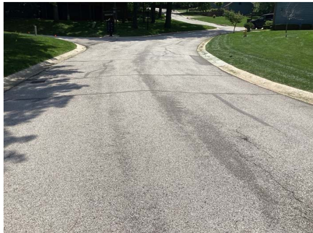
Pavement overview at Lakeside Dr, note various cracks and repairs
