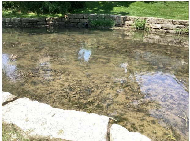
Sediment accumulation at north pond
