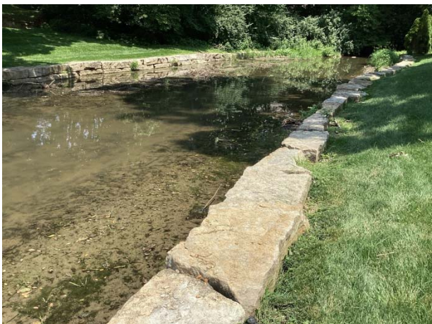
Shoreline erosion and sediment accumulation at north pond
