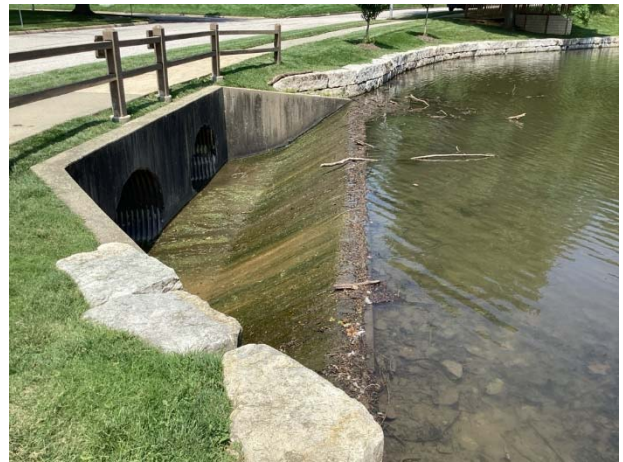
Concrete spillway at south pond
