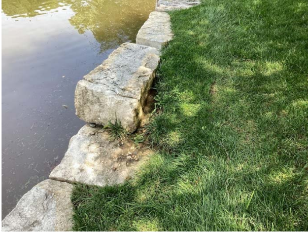
Erosion at wall backside
