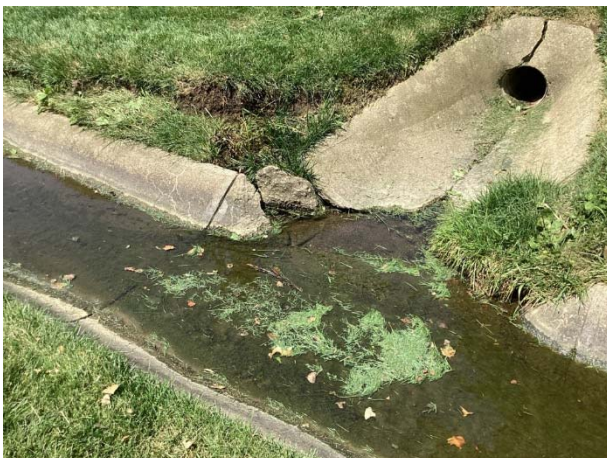
Concrete channel deterioration and erosion
