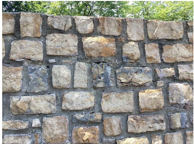
Mortar and stone deterioration
