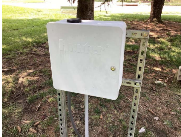
Irrigation system controller
