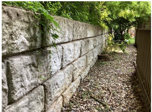
Concrete retaining wall behind east side homes on Lakeside Dr
