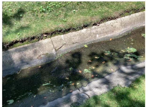
Concrete channel cracks and spalls
