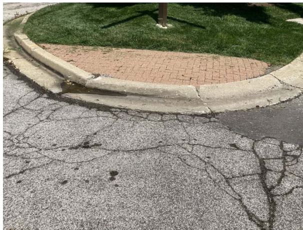
Concrete curb and gutter deterioration
