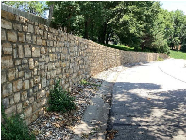
Mortar-set retaining wall at Seaport Circle
