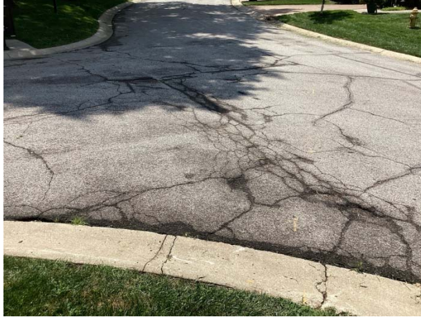
Alligator cracks and pothole formation
