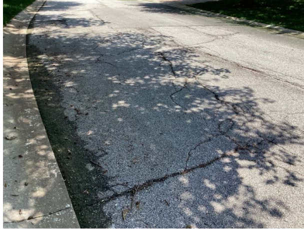
Edge deterioration, cracks and patches at Seaport Circle
