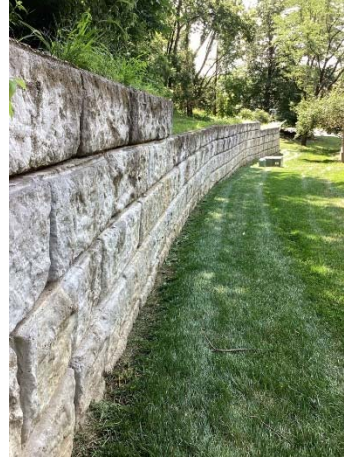
Minimal amount of wall lean noted towards southern end of wall
