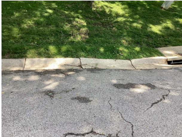
Concrete crack and settlement
